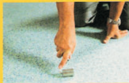
⑭ Final roll and damp sponge finished seam
