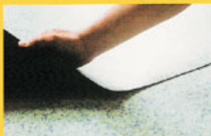
⑤ Overlapping sheets for double cutting
