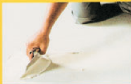
⑧ Turn back the 2 pieces to apply standard adhesive
